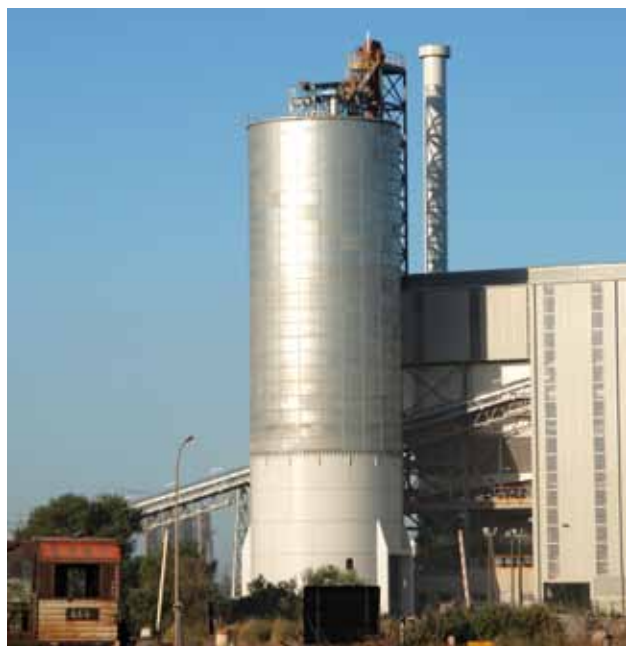
3.300 m 3 silo for cement delivered in France, 2009.
